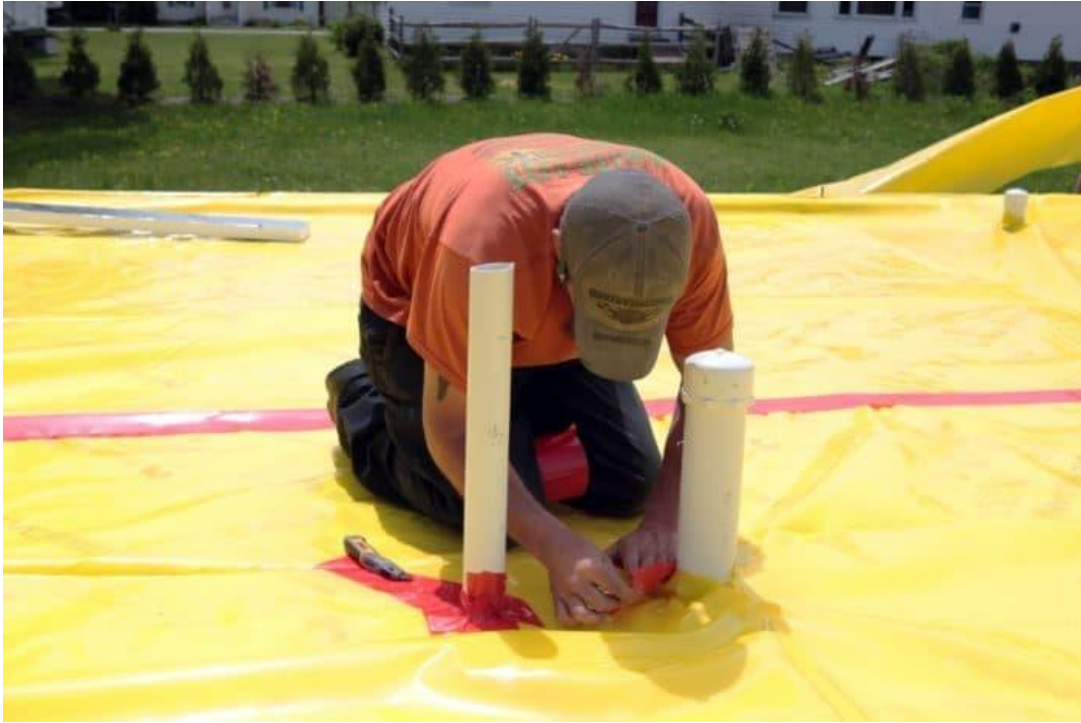
All vapor barrier seams and penetrations are sealed with tape
