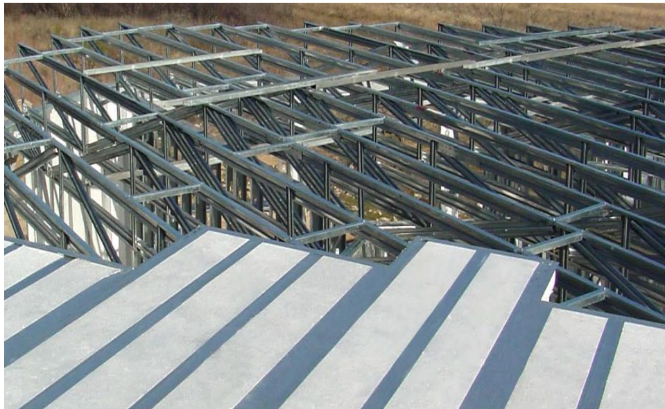
Above are ThermalSteel™ Panels married to metal trusses
