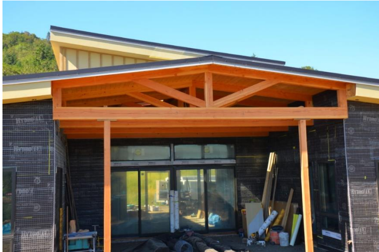
Big timber trusses from second growth forests
