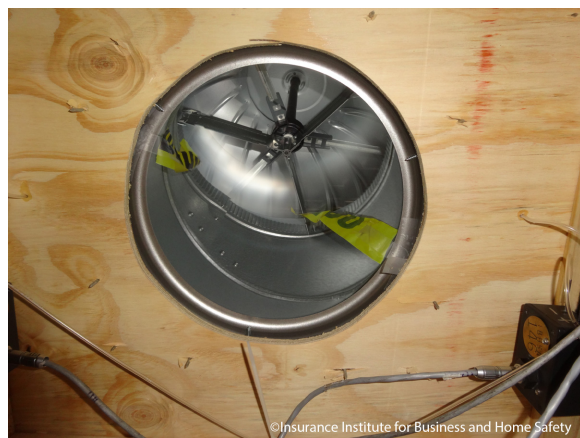
Figure 17. As indicated by the action of the ribbons, the ridge vent (left) and turbine vent (right) were consistently outlet vents.
