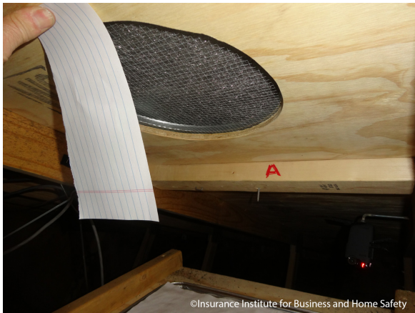
Figure 15. As indicated by the action of the ribbons, on the windward side of the building, the off-ridge through-roof vent (left) and open-eave vent (right) were inlet vents.
