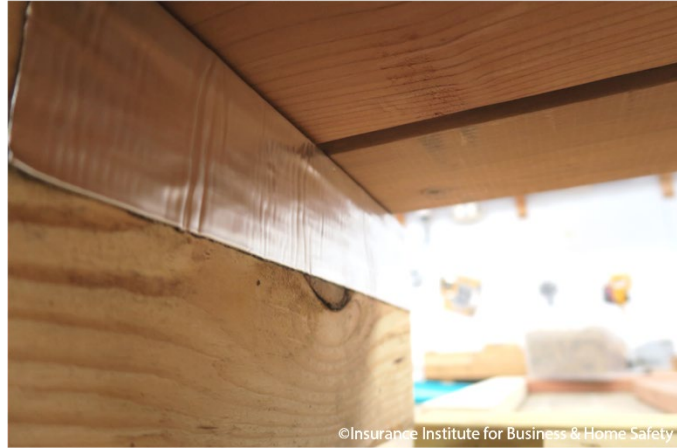
Figure 8.1. Placing foil-faced tape on the top and sides of a deck joist has been shown to reduce vulnerability of deck boards, especially combustible products like cedar or redwood. Photo: IBHS.
