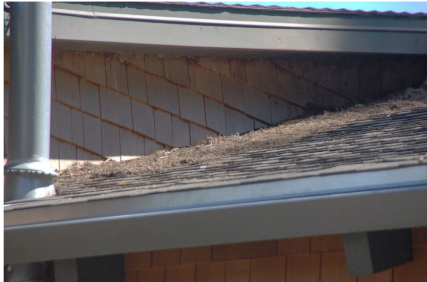
Figure 6.1. Complex roof showing roof-to-siding junction where pine needle debris has accumulated on top of asphalt composition shingle roofing (a Class A fire-rated covering), adjacent to wood shingle siding. The vulnerable component of this roof is the siding, should the pine needle debris ignite. Photo: Stephen L. Quarles
