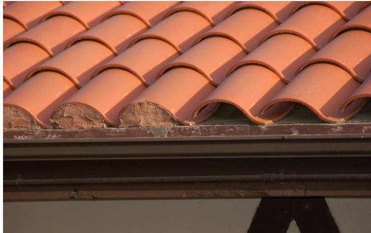
Figure 6.6. Use of a mortar mix to provide an effective “bird stop” at the edge of this barrel style roof (this photograph was taken during a retrofit project while the work was in progress). Photo: Stephen L. Quarles
