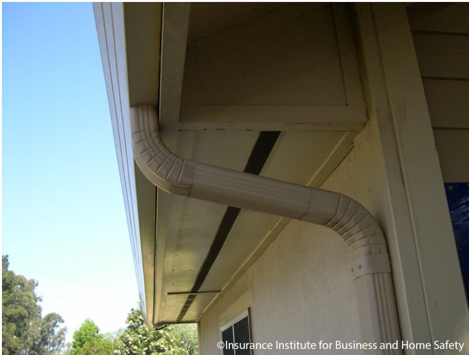
Figure 2. A strip vent located in the soffit of a building that used soffited-eave construction.
